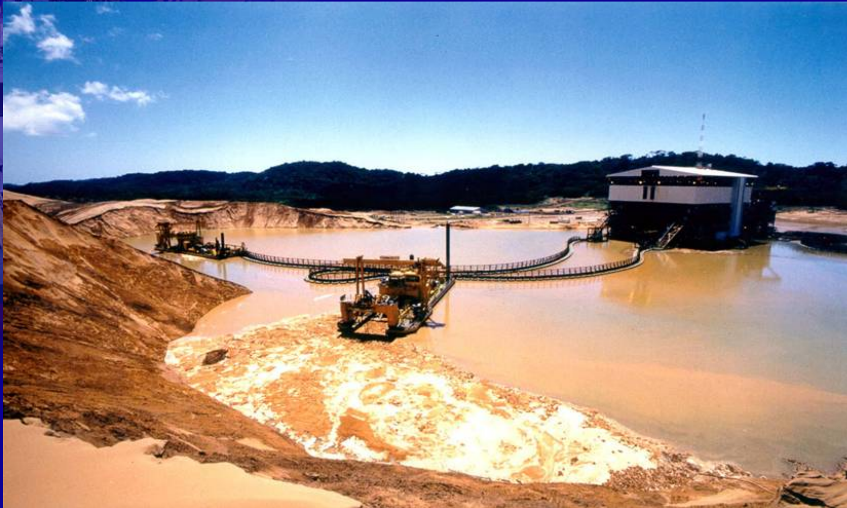
Dredgers at work for the heavy minerals mining industry (South Africa)
